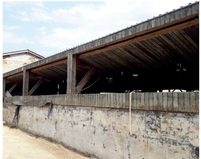
Photo 20 - Installation de volets
